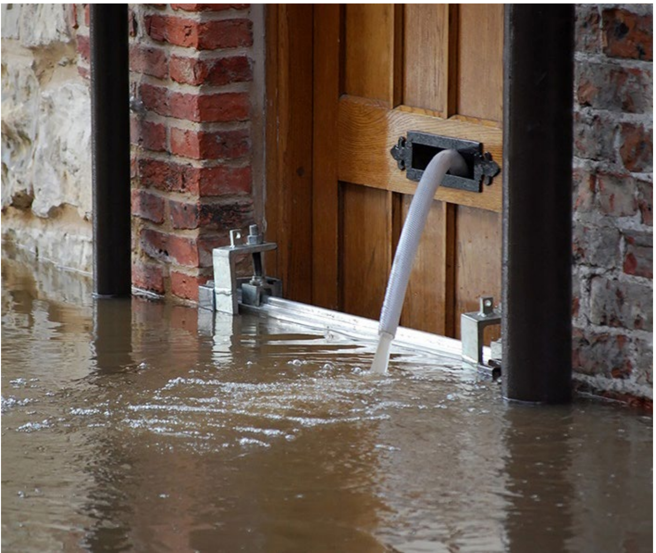
Figure 5-1. Floodwater being pumped from a property in Gloucester.
